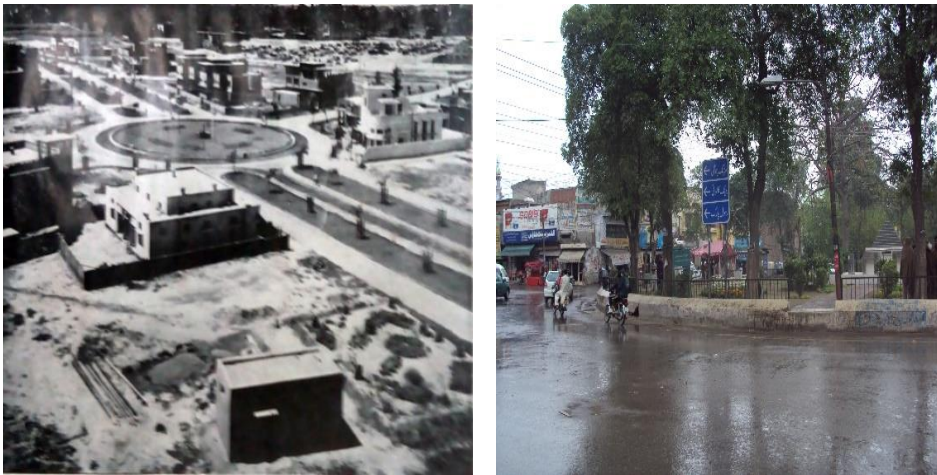
Figure 5. (Left): Samanabad first round-about, development underway (Right): Samanabad first round-about at present
