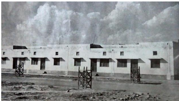
Figure 3. Trees are being planted along the Roads (Source: LIT)
