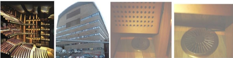
Figure 2. Internal view of main hall, external supply and extract openings, supply grills under seats
