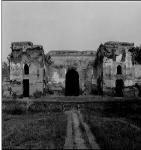
Figure 4. Jahangir's tomb destruction and encroachments
