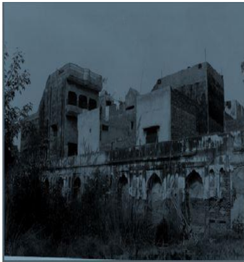
Figure 5. Encroachments along Jahangir tomb's boundary wall
