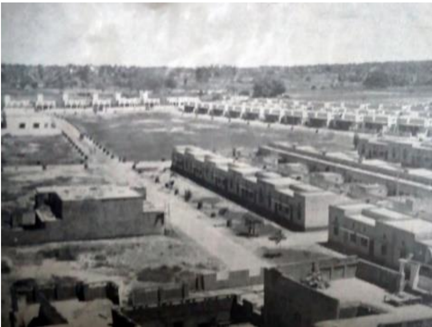
Figure 4. Samanabad quarters under-construction (source: LIT)
