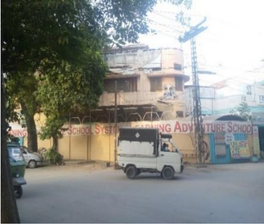
Figure 7. The same house in 2015 (Source: LTI)
