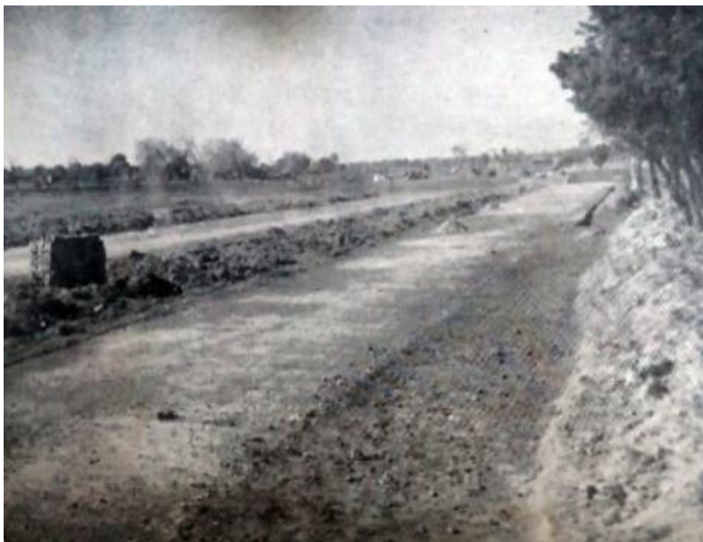
Figure 2. Preparations for construction (source: LIT)
