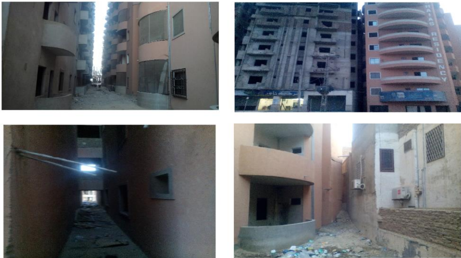
Figure 1. Existing insufficient setback area and openness
