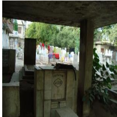
Figure 4. An enclosure roofed for the graves of the same family.
