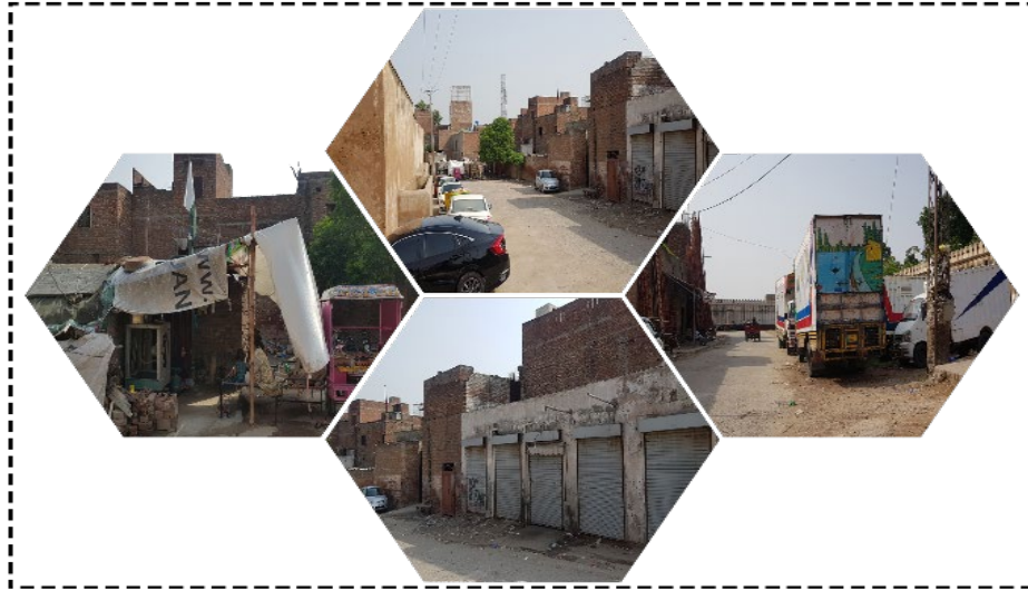
Close View of Encroachment at Shalimar Gardens
