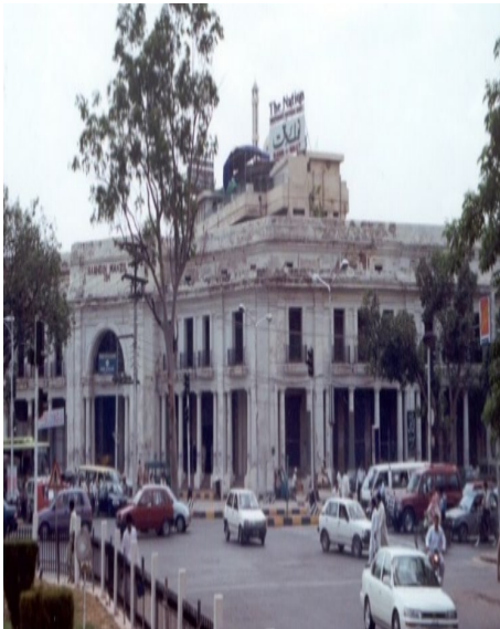
Figure 6 Shah Din Manzil, Before Renovation
