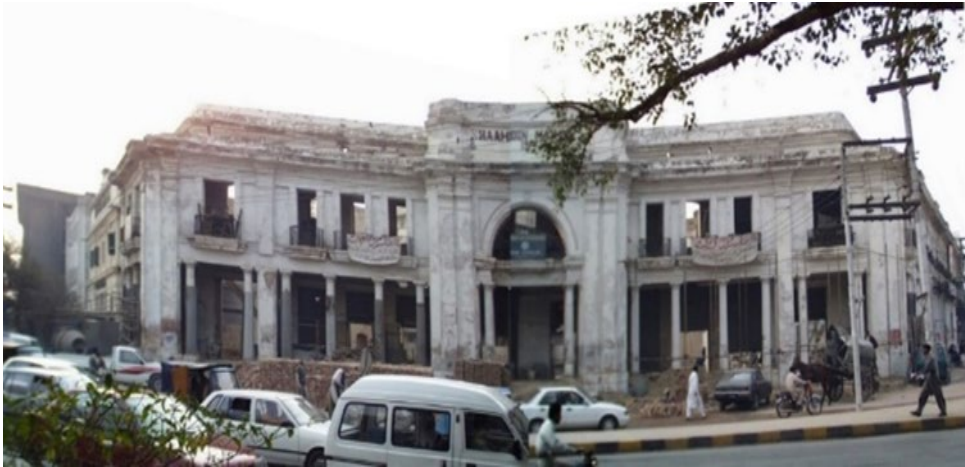
Shah Din Manzil, Before Renovation
