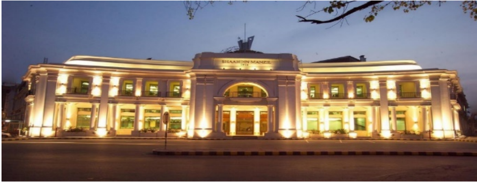
Figure 5 Shah Din Manzil, After Renovation
