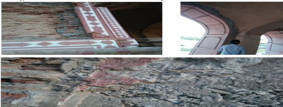
During Restoration Work in 2020 Ordinary Portland Cement was Used
