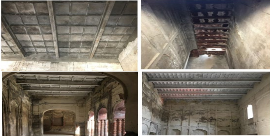
Ceiling Condition of Different Areas
