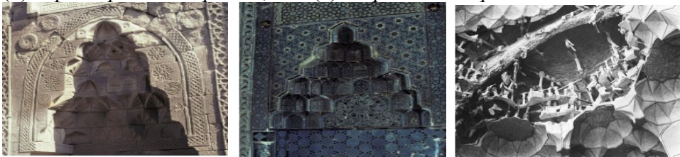
Muqarnas Construction in Three Different Ways: (a) Corbelled Muqarnas; (b) Superimposed Muqarnas; and (c) Suspended Muqarnas
