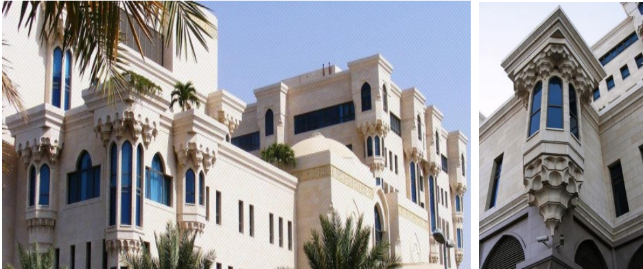
(a) Muqarnas Details of International Medical Center Jeddah, Saudi Arabia ; (b) Muqarnas Details on the Balcony of International Medical Center, Jeddah
