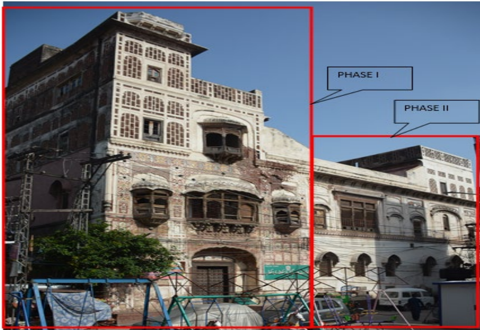
Haveli Naunehal Singh Showing Two Phases of Construction with Off-centered Entrance, Lohari Gate, Lahore
