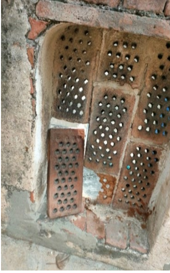
Figure 6 Traditional Style Brickwork in the Building
