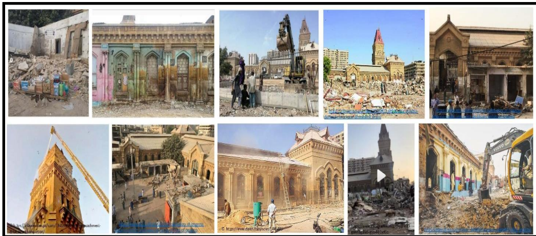
Various Images Show Deliberate Man Made Vandalism By Anti-Encroachment Drive In 2019, Section Shows Internal Space Layout,
