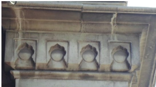
Detail of the Top Portion of the Pillar Frieze of Dentils Under the Trefoil Pattern
