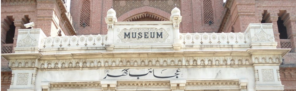
Parapet of the Façade
