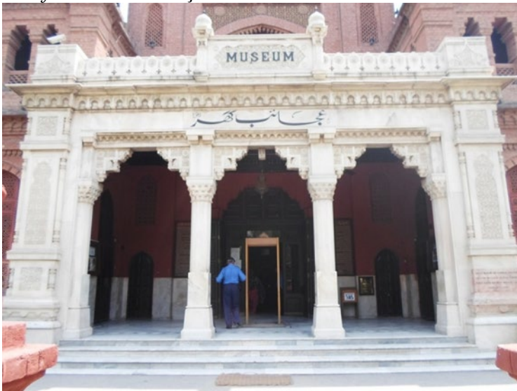
Front View of the Marble Façade
