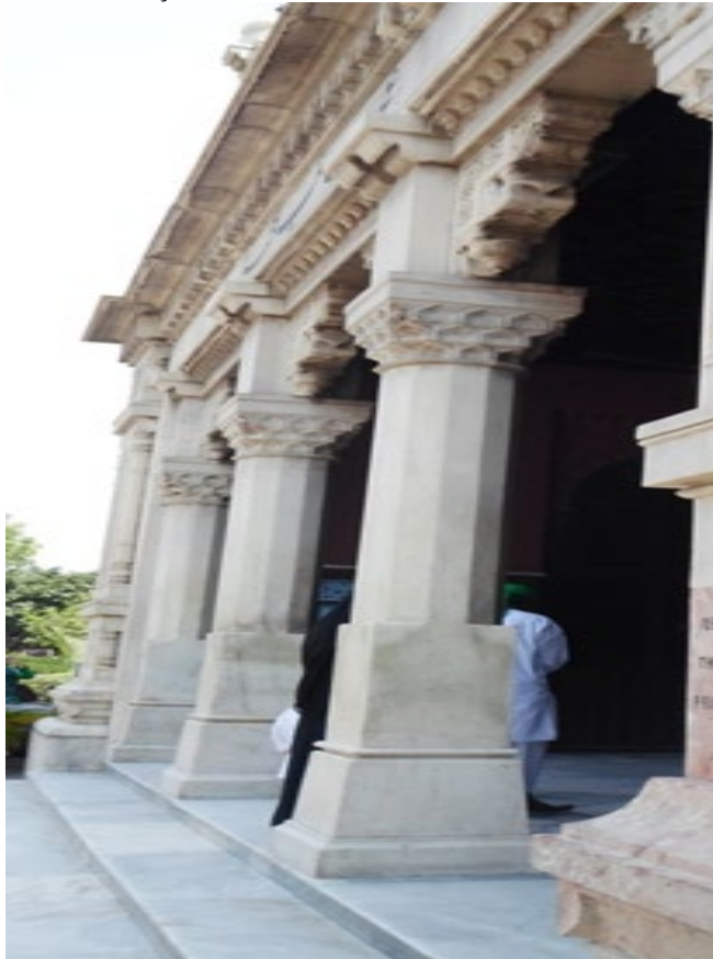
Columns of Marble Façade
