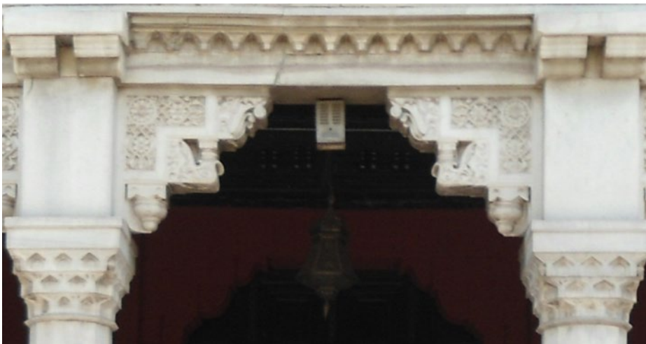
Corbelled Arch of the Façade
