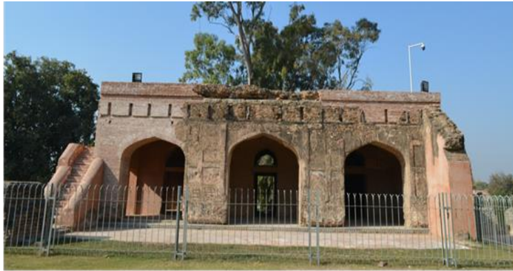
Existing Condition of Baradaris in Second Terrace
