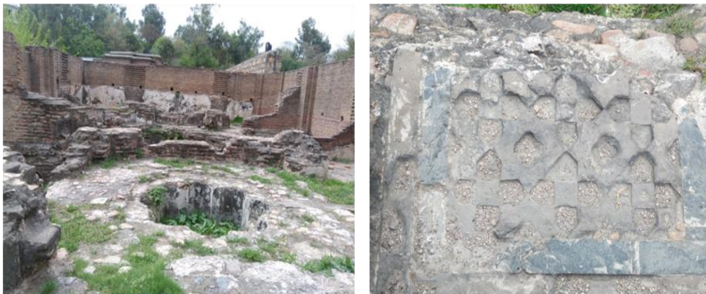
Existing Condition of the Hammam and the Geometric Patterns on its Floor
