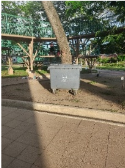
Figure 16 Pavement made from Eco-bricks (Recycled Plastics)
