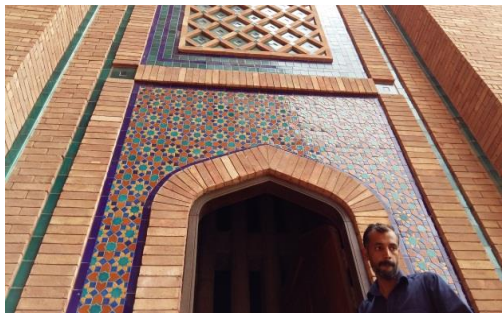
i: View of the Blue Tile Work of Minaret
