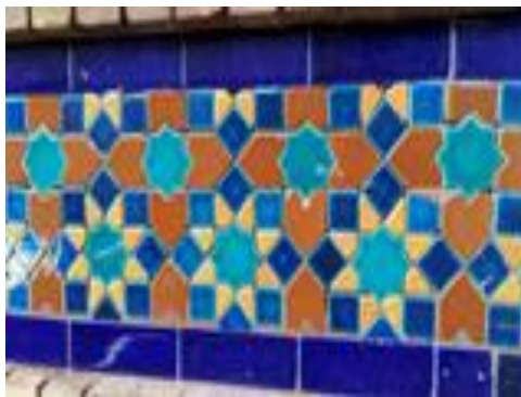
ii: View of the Blue Tile Work of Minaret
