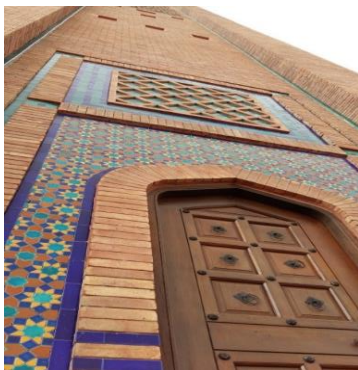
i: View of the Blue Tile Work of Minaret
