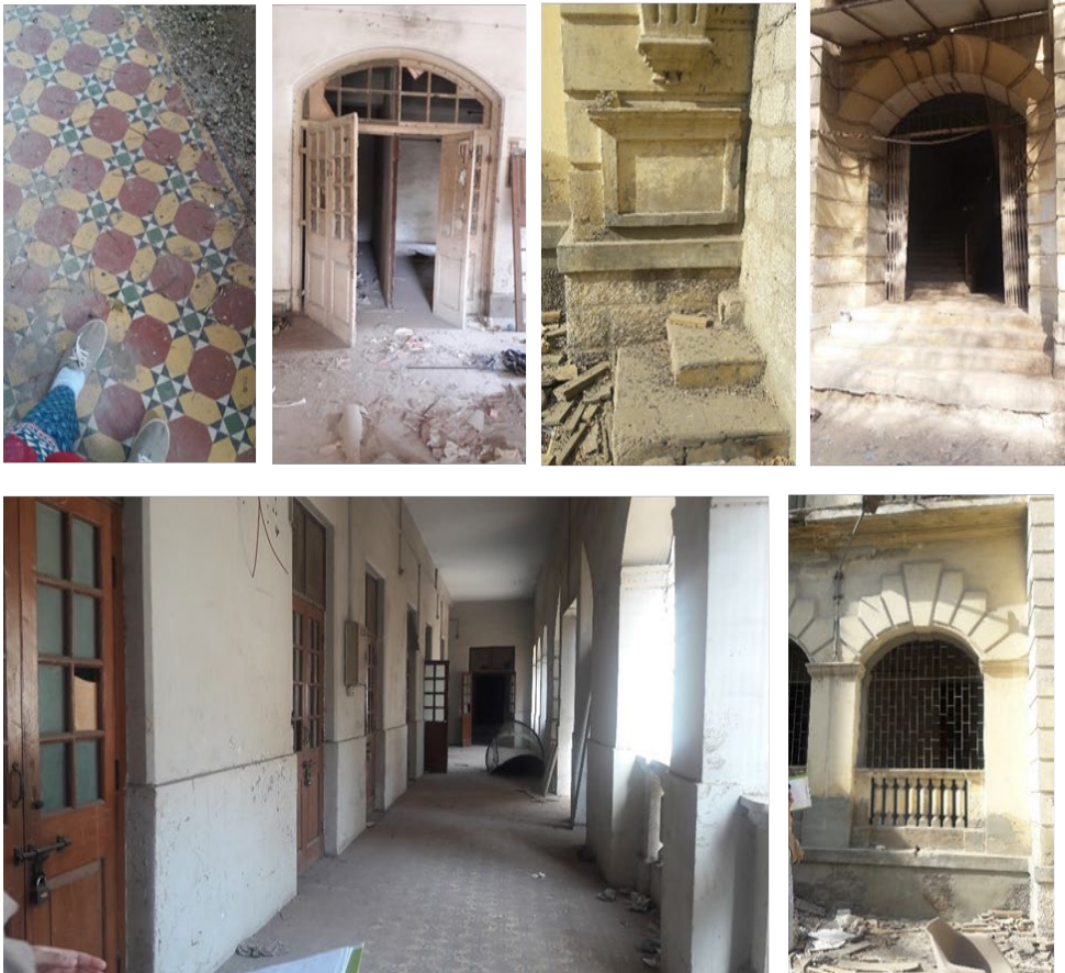
Photographic Documentation of Doctors' Mess – Detailed Images of the Interior of the Building
