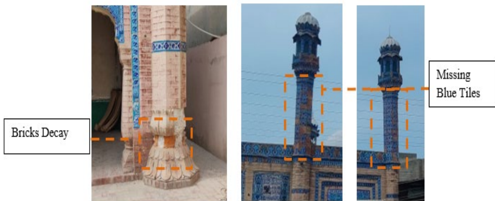
Decay of Materials on the Outer Façade of Jamia Masjid Akbaria
