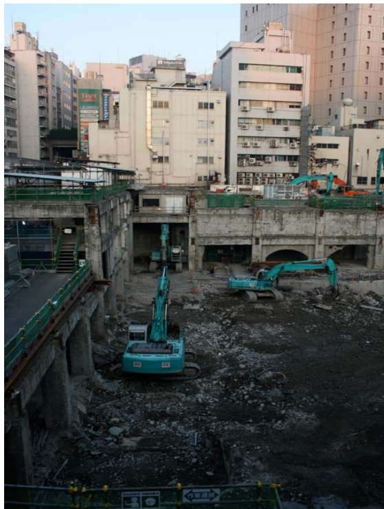
Excavating Machines for the Expansion of Shibuya Station
