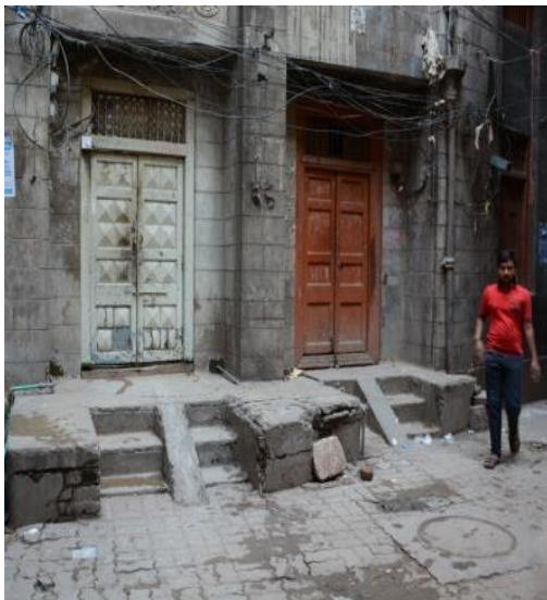
Deck outside a House
