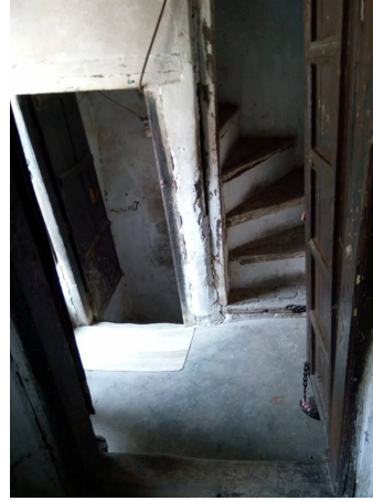
Fig-13. Staircase from the south wing
