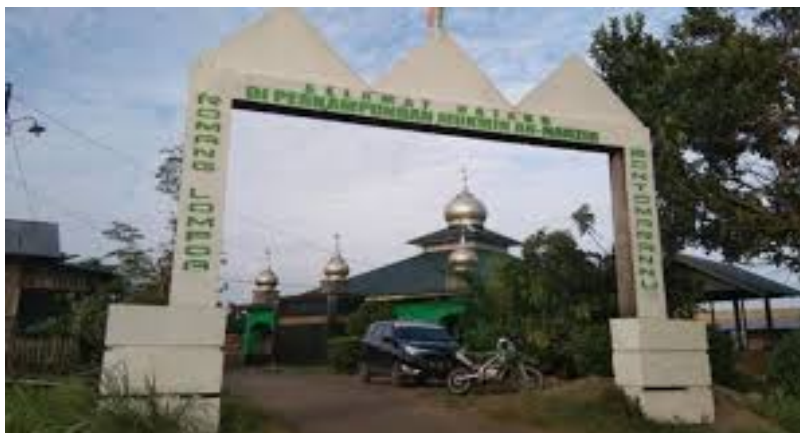
Figure 2. The Mosque of An-Nadzir Community 43
